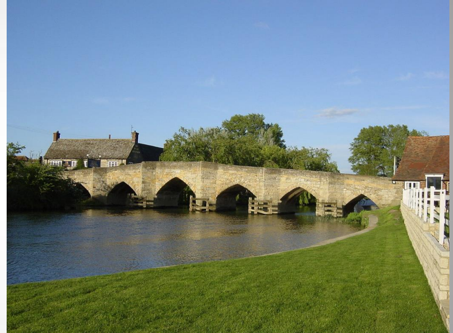
New Bridge (13 th century)
