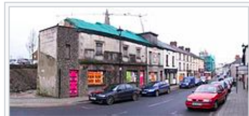
The currently closed "The First and Last" Pub, next to the closed Omagh railway station , in County Tyrone , Northern Ireland . ↗
