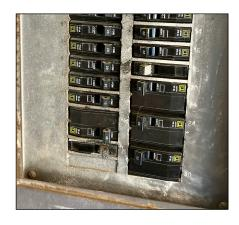
If your electrical box is full (above), you have few options. Upgrading service to the house, adding auxiliary box and then 240v circuit will be very expensive. With unused slots in the box, (above center) you can add 240v outlet or direct wire a charger.
