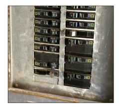
If your electrical box is full (above), you have few options. Upgrading service to the house, adding auxiliary box and then 240v circuit will be very expensive. With unused slots in the box, (above center) you can add 240v outlet or direct wire a charger.
