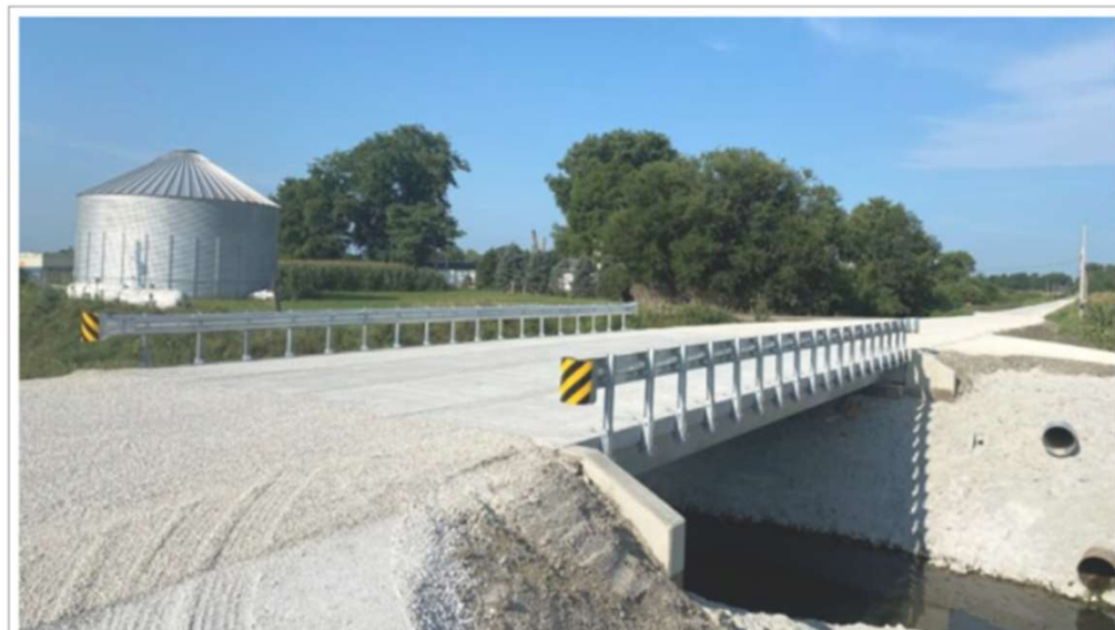
Champaign County's press-brake tub girder bridge has a 100-year total bridge service life for an upfront cost that is less than the concrete beam option.
