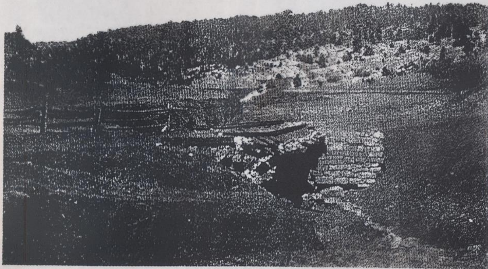
Near View of the Strategic Bridge in the Lower Battlefield in the Apache Canon. (From one of the author's photographs.)
