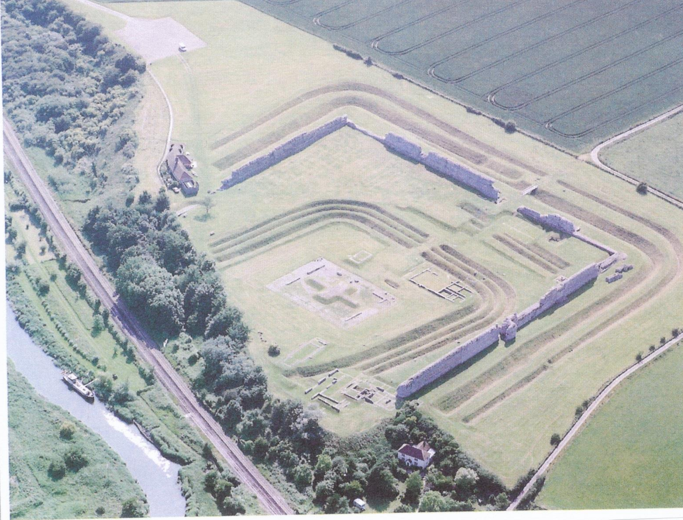
60 (above) Aerial shot of the fort at Richborough, Kent. In the centre of the fort the cross-shaped foundation is the base of a four-way monumental arch, built towards the end of the first century AD. Surrounding this is a square enclosure constructed in the early third century, forming a military stronghold around the by-then ruined arch that was probably used as a look-out tower. The final major phase of defensive architecture is the tall flint-built wall of the Saxon Shore fort enclosing the whole site, built c. AD 275.
