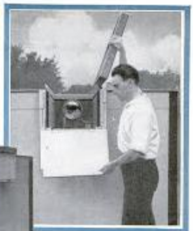
Peltier shows how the lid is lifted from the telescope well. The inside of the structure is painted a dead black to minimize light reflection
