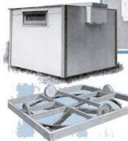
Exterior of the midget observatory, and its base framework with circular track. Wheels are from a child's merry-go-round
