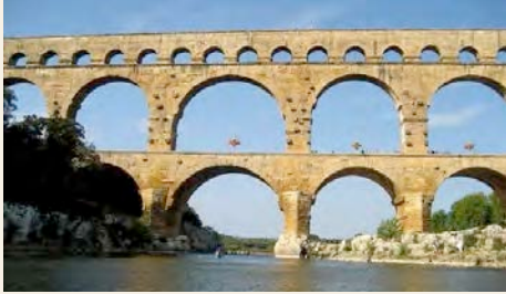
Roman aqueduct near Arles France, one of the best preserved examples of Roman hydraulic engineering
