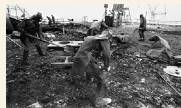
Workers removing radioactive materials from the site
