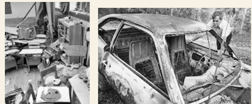
Left: Damage caused by a presumed dynamite blast at Midway Elementary School in Kanawha County, W. VA.
