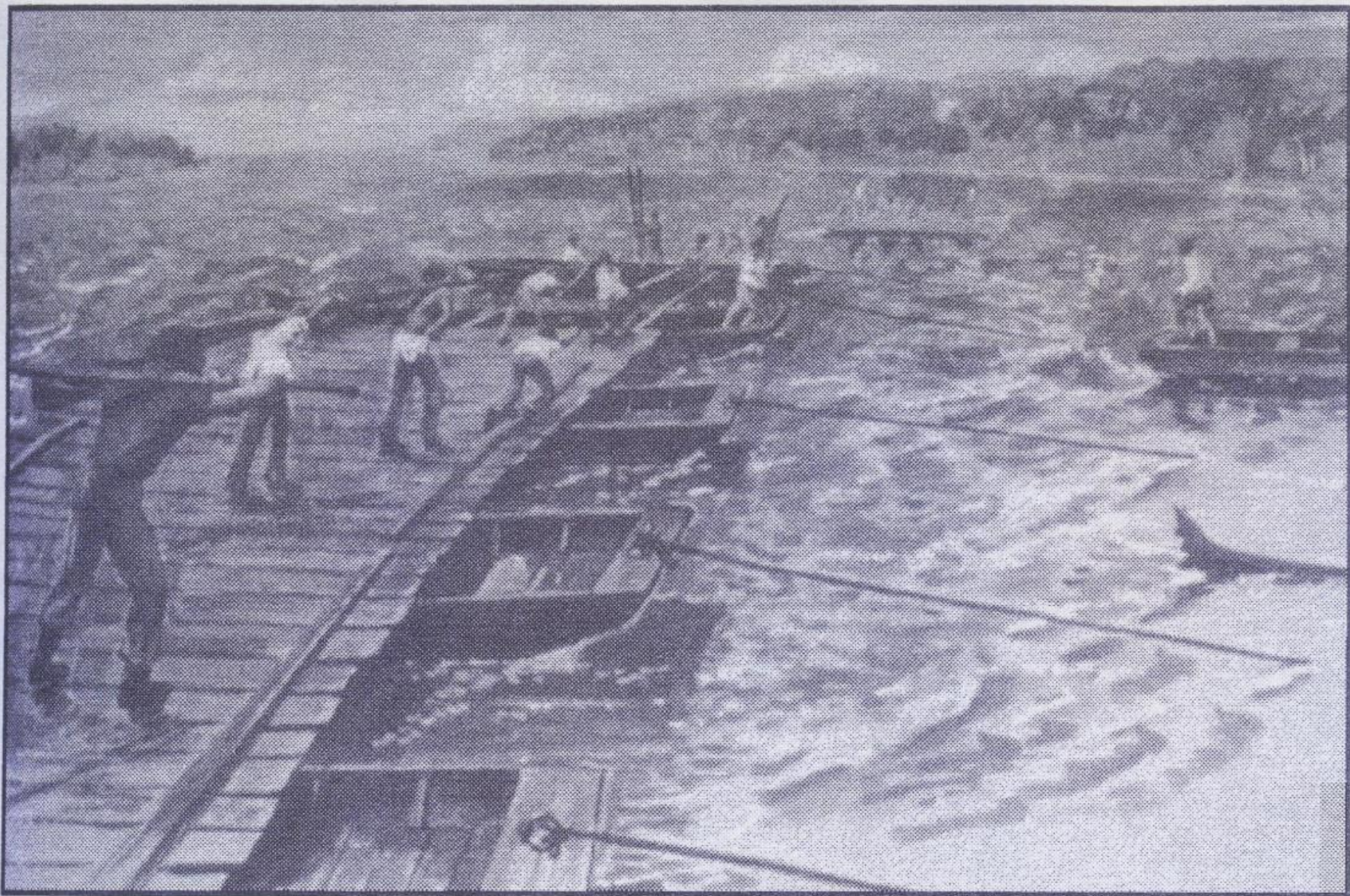
Major Harman builds a pontoon bridge at Falling Waters, using lumber from demolished Williamsport warehouses which had been hauled downstream.
